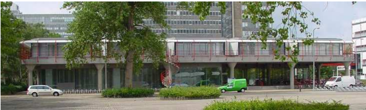
Embedded Systems Institute (ESI)
