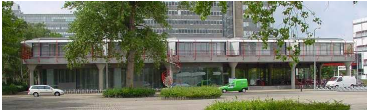
Embedded Systems Institute (ESI)
