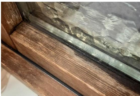
Example of condensed water in a bath room at 7°C, -17°C outside with an old double glass window
