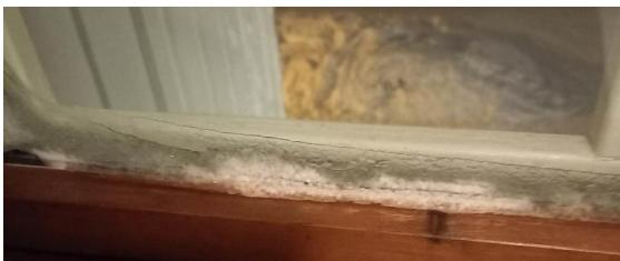
Example of frozen condensed water in an unheated room with an old double glass window
